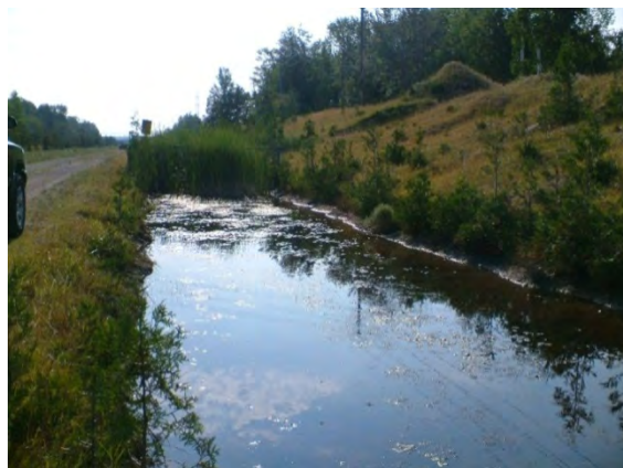
South Railway Ditch
