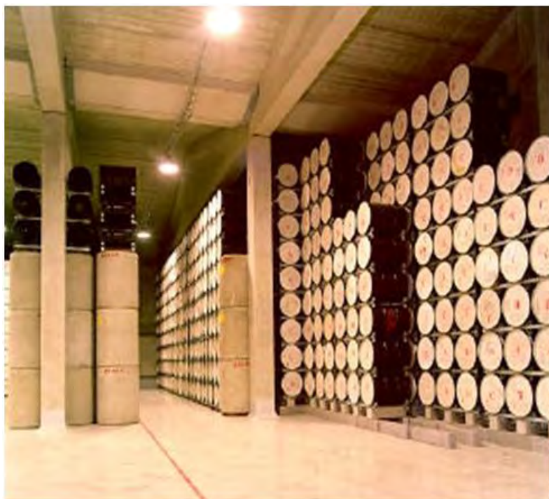
Figure 4.1: Photos of the long-term L&ILW storage building and containers at COVRA in Netherlands. Each building has a capacity for about 5000 m 3 of waste, has 40-cm thick concrete walls and a design life of 100 years.
